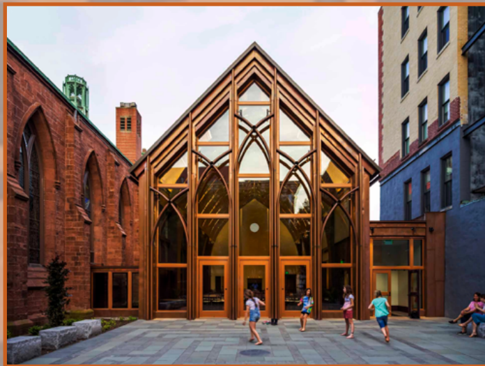
The Pavilion at Grace Episcopal Church, Providence, RI
